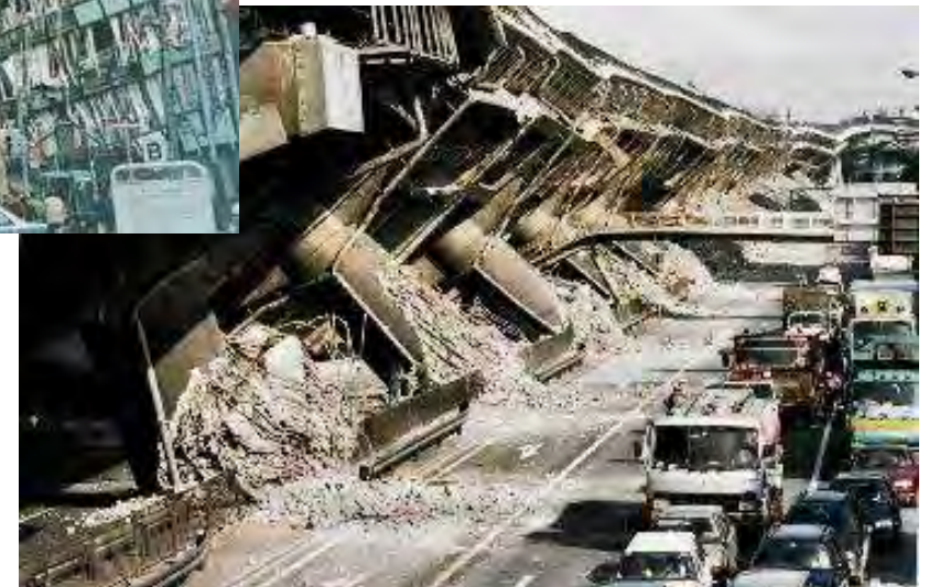
Collapsed viaducts of an expressway
